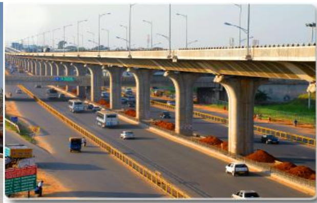
b. Elevated toll road access.
