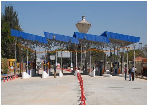
a. Toll collection area in the Electronic city.
